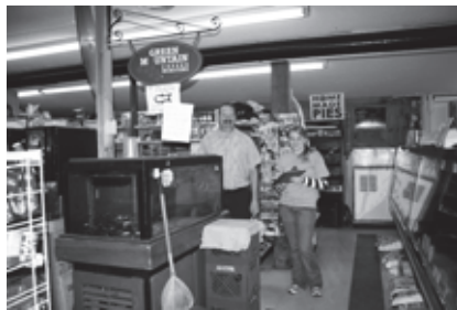
Steve Berger saved Northwood Market's live bait tank refrigeration system.
